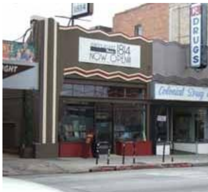
An appropriate paint scheme can showcase a building's original architectural features.
