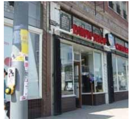
Individually cut channel letters, mounted to a canopy, allow for the transom window to remain open.
