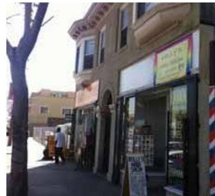
Many upper-floors on Jefferson Boulevard commercial structures are accented by dual bay windows.
