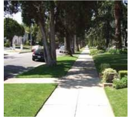
Sidewalk widths, parkway landscaping and sidewalk score patterns should all be preserved.
