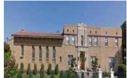
Sister Servants of Mary Convent located at 2131 W 27th Street, built in 1931.
