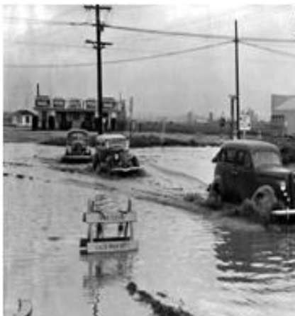
Flooded Jefferson Blvd. near Centinela 1941
