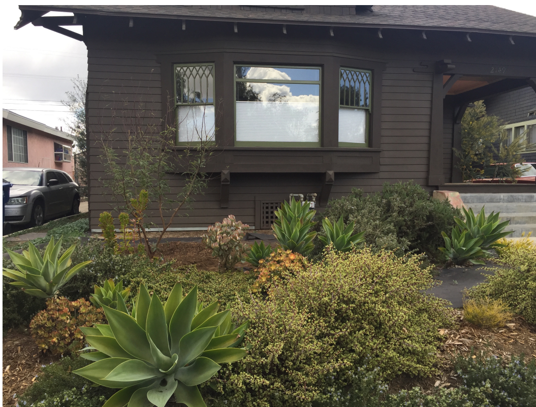
The windows after restoration.
