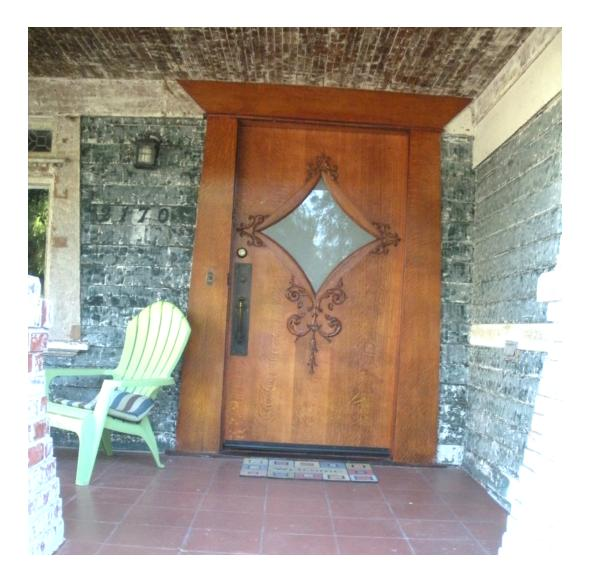
This house is in the process of being stripped to reveal its original color scheme. The body was stained dark bottle green, the trim was a cream color and the sashes were painted black. The door and its frame were stained. The porch ceiling was typically finished (not painted).
